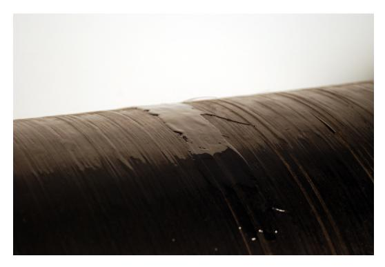
▲ There should be no indentations or low spots in the repaired area, which should extend slightly above the original surface of the cylinder.
