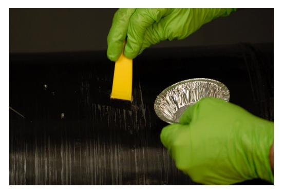
▲ Apply resin to damaged area, ensuring that resin is worked fully into any damage. Allow to dry, following manufacturer's instructions.
