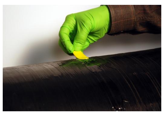
▲ Continue applying resin until the gap left by delamination is completely filled. Allow to dry, following manufacturer's instructions.
